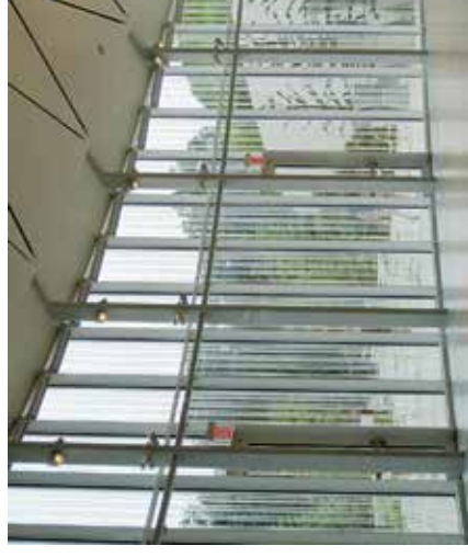
Glass walls and doors at the Brooklyn Botanic Garden's Visitors Center include a custom fritting pattern that meets bird-friendly criteria. Monitoring for collisions after the building opened indicates that the design was successful. Photo by Christine Sheppard, ABC
