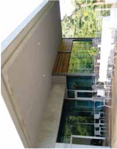
Overhangs block viewing of glass from some angles, but do not necessarily eliminate reflections. Photo by Christine Sheppard, ABC
