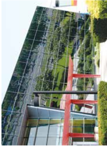
Reflections in this angled facade can be seen clearly over a long distance, and birds can approach the glass from any angle. Photo by Christine Sheppard, ABC
