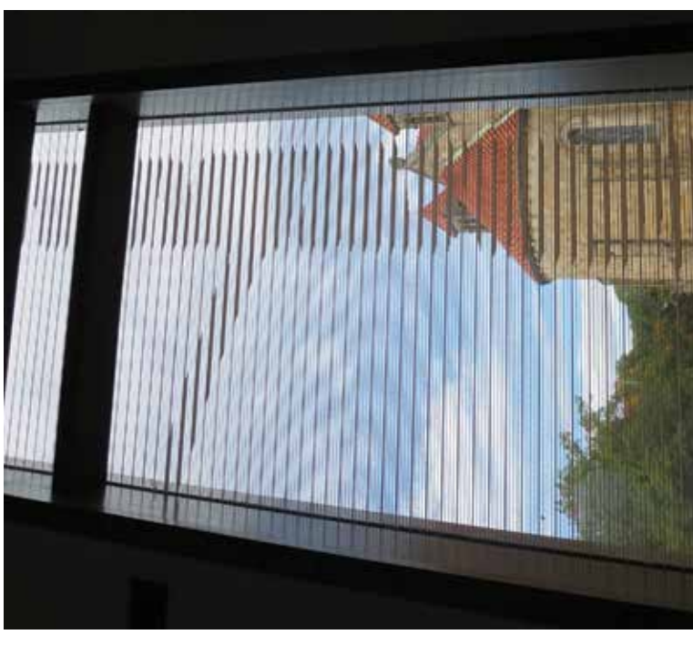
A custom frit pattern was designed by Ennead Architects for Vassar College's Bridge for Laboratory Sciences building. Elements of the pattern occur on two separate surfaces, increasing visibility to birds in flight, who will see a constantly changing pattern that may appear to move. Photo by Christine Sheppard, ABC
