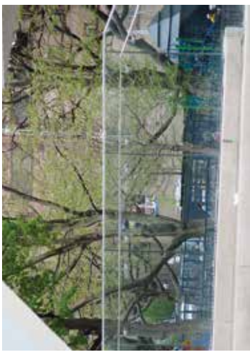
Transparent handrails are a dangerous trend for birds, especially when they front vegetation. Photo by Christine Sheppard, ABC
