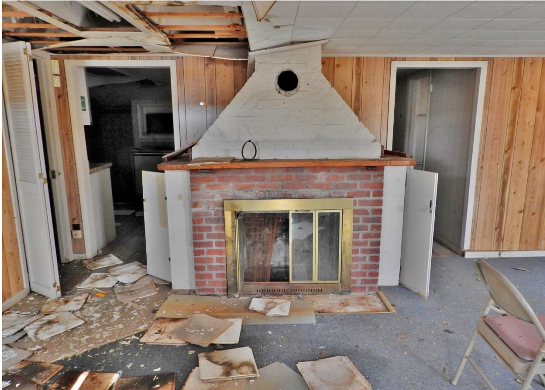
19. Facing west in main block.
