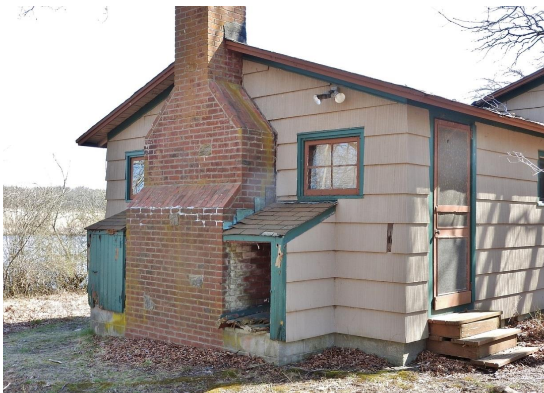
14. Facing southeast toward north wing.
