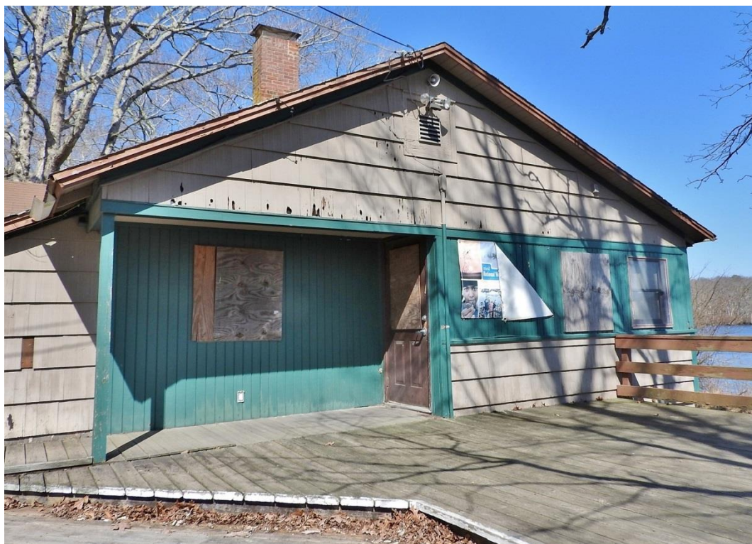
8. Facing northeast toward south elevation of main block. Full-height green siding installed in 1987 over location of original front door.
