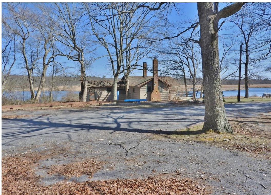
4. Facing southeast toward Cabin across service road.
