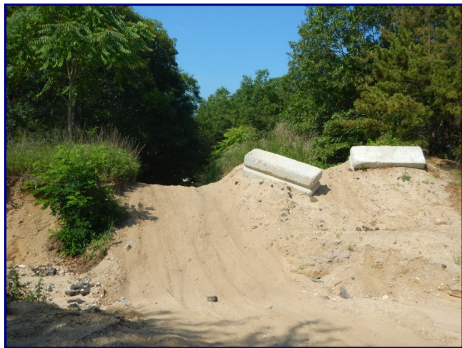
Damage and erosion caused by illegal ATVs
