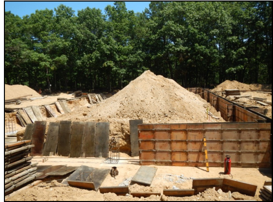
Camp Wauwepex — Rebuilding dining hall that burned down
