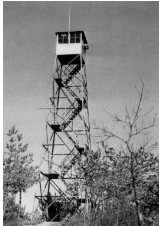
Flanders Hill Tower, 1946 Photo Credit: NYS DEC
