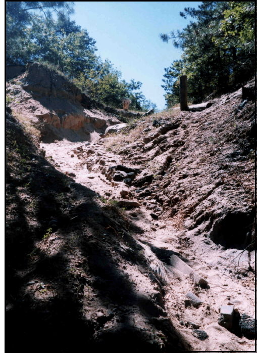
Off road vehicle erosion is severe in certain locales. This scene from a September patrol shows the dramatic grade drop that can occur.
