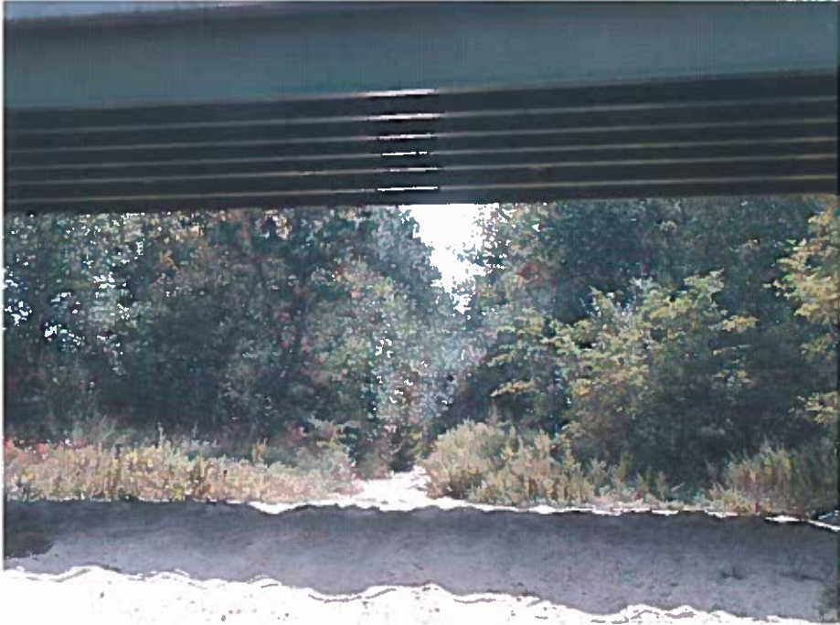
View of existing dirt road where it narrows west of the CR 111 overpass
