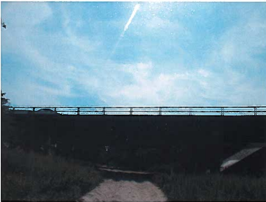
View of CR 111 overpass
