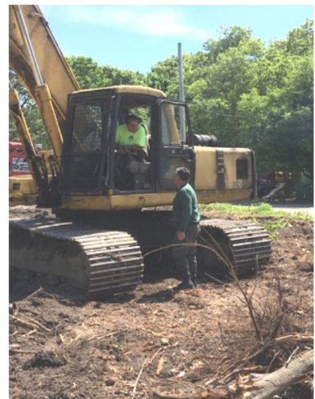
Officer Jim Mazzio checks a backhoe operator clearing land in Flanders
