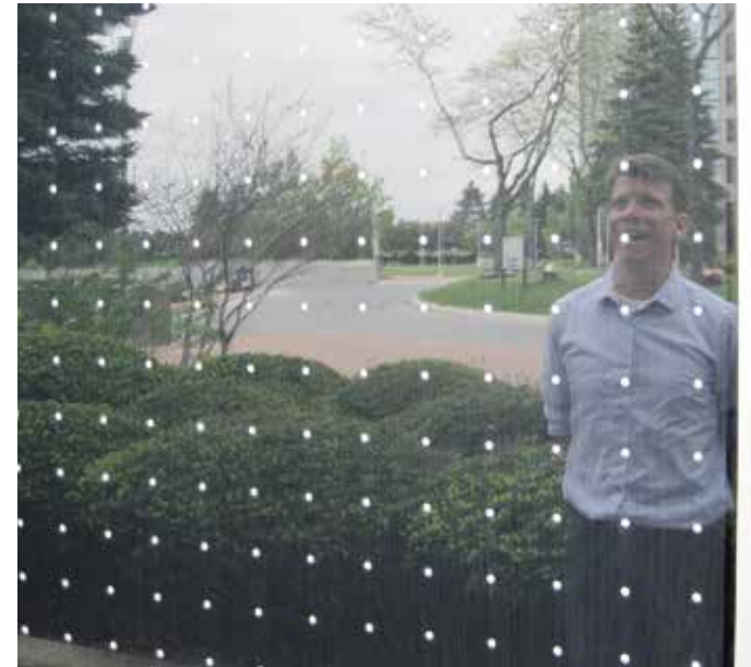
The Consilium Towers, a mirror-glass complex in Toronto, once killed thousands of birds each year. After being taken to court, its owners retrofitted the lower 60 feet of glass with a Feather Friendly dot pattern that has greatly reduced bird mortality.
