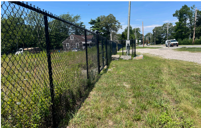
Fig 3 Existing fence set back from road.
