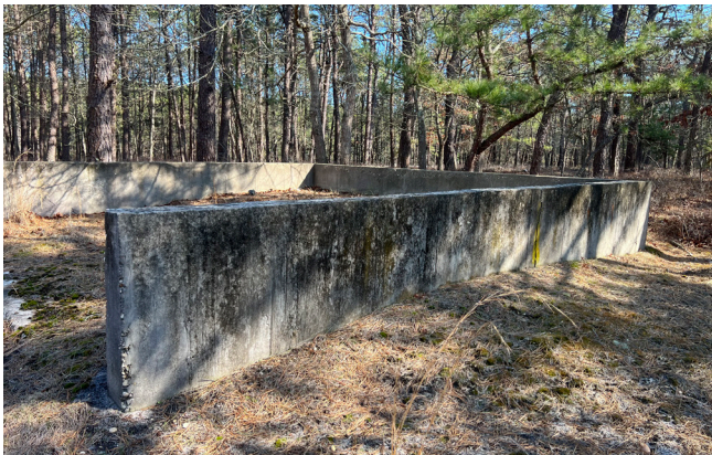
Fig 3 Existing concrete foundation on site
