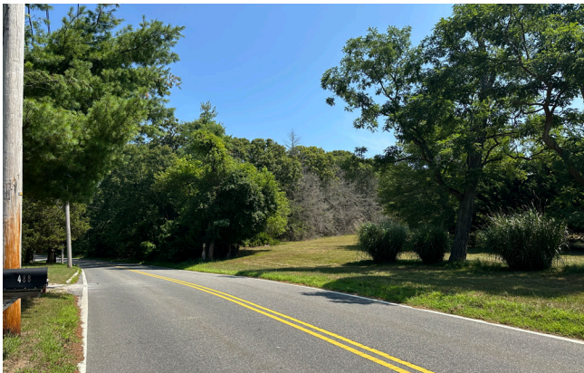
Fig3 View of road leaving DEC check-in station.
