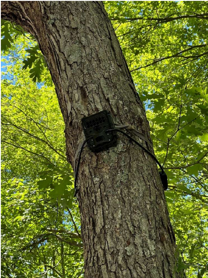
Surveillance camera installed on Ashton Road in Middle Island
