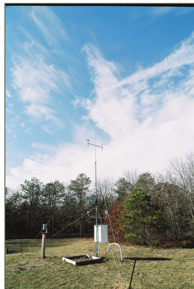
Eastport Fire Weather Station
